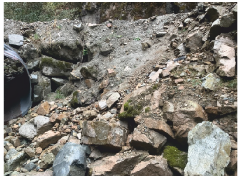
Downstream left riprap
