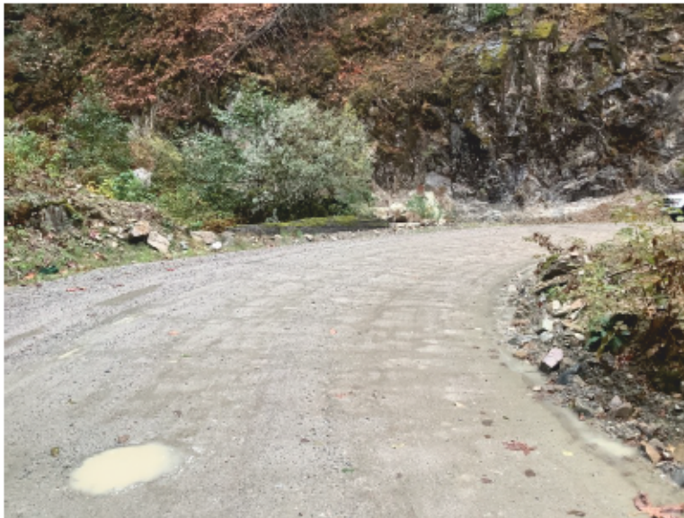
Approach from Right Bank when facing downstream
